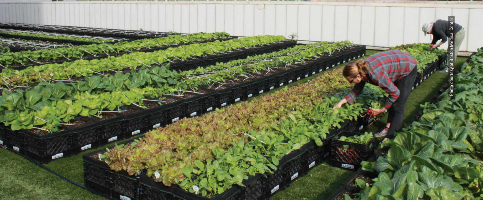
Boston Medical Center's new rooftop farm project has transformed the once-barren roof of its power plant building, further exemplifying the hospital's sustainability efforts.
