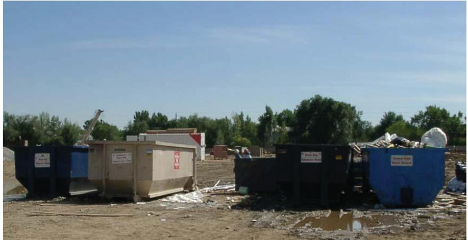
Photo credit: Boulder Associates Architects, 2003. On-site roll-off dumpsters are used to separate and collect construction demolition and debris.
