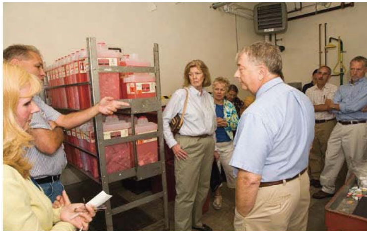
Sharps containers in central hazardous waste accumulation area at the Albany Medical Center's South Clinical Campus.
