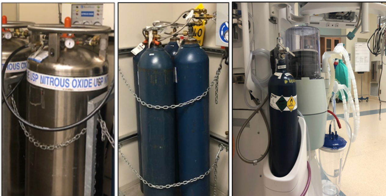
Left to right: Cryogenic tanks in tank room, H-cylinders in tank room, and E-cylinder on anesthesia cart.
