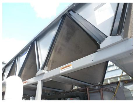
Figure 25: Chiller-1 Condenser Coils
