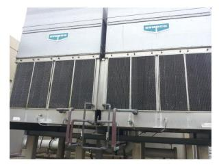
Figure 7: Evapco Cooling Towers
